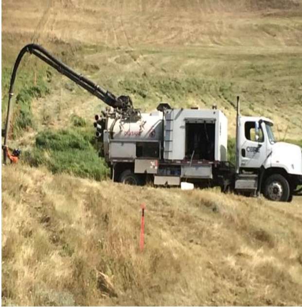
686 + 500 – 687 + 300 Hydrovac – slurry pit and signage
